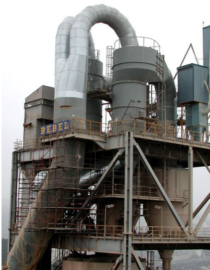
Alhandra plant (kiln 7)
