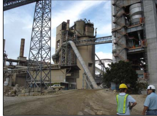
Fig.4: Existing raw meal silo of Holicm Costa Rica.
